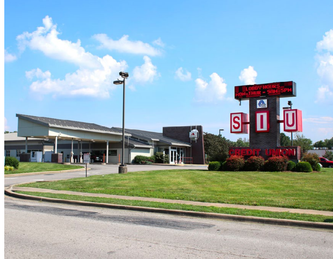
SIUCU’s headquarter branch in Carbondale, Illinois. Image: SIUCU
